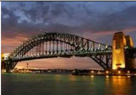
Sydney Harbour Bridge
