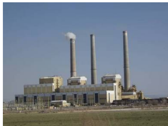
Figure 31. Coal-fired electric power plant.
